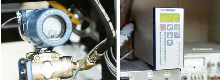
Figure 3.1. Pressure transmitter and digital valve controller.
